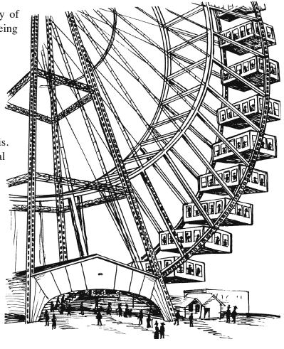
No steel company could handle the manufacturing job alone. Ferris had to contract with a dozen companies to produce the bars, trusses and girders, which were meticulously planned to fit together like giant Tinkertoys when assembled at the site.
